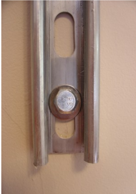
The left photo shows proper lag screw installation
